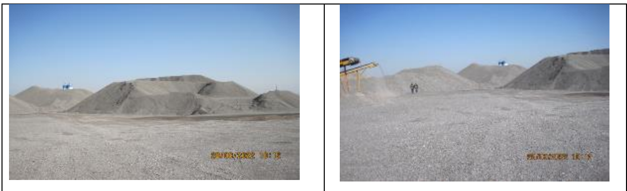
Figure 21 Preparation of gravel material for the production of concrete and asphalt
