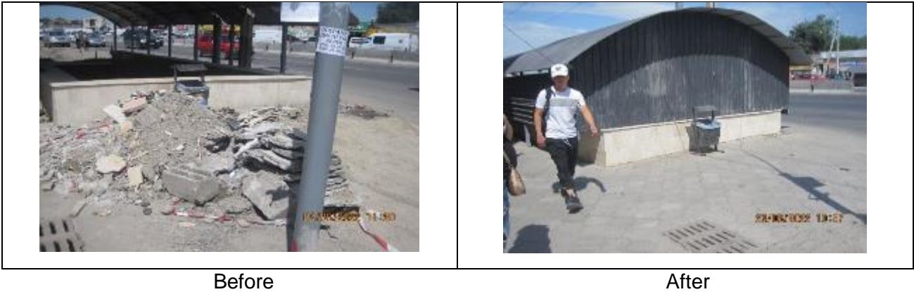
Figure 57. Construction waste near the underpass under construction in the center of the Sokuluk.
