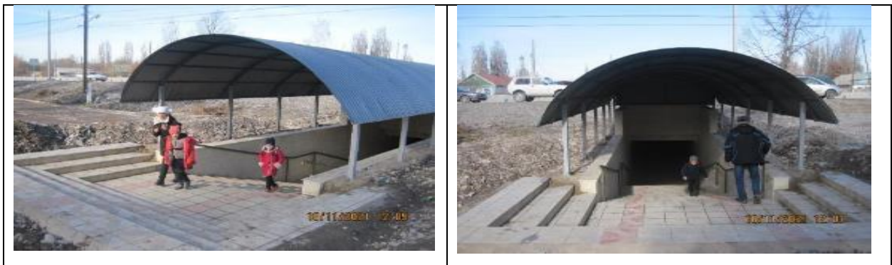
Figure 10 Underpass in the Novonikolaevka
