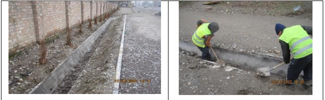
Figure 29 Cleaning of side culvert ditches
