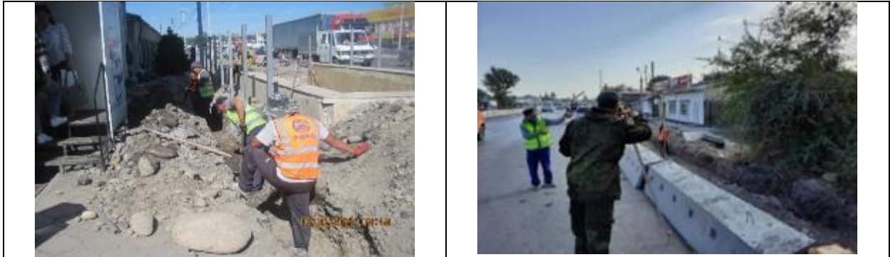
Figure 4 Installation of side culvert ditches
