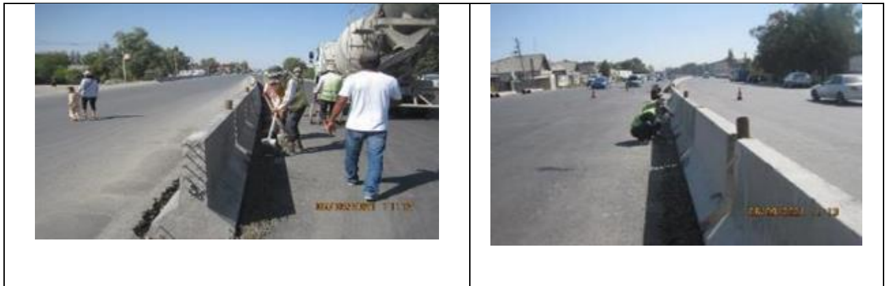
Figure 30 Works on concreting cut on passages between parapets
