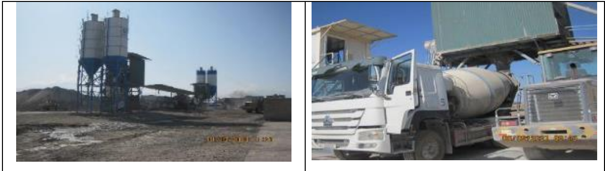
Figure 22 Filling the concrete mixing machine with concrete
