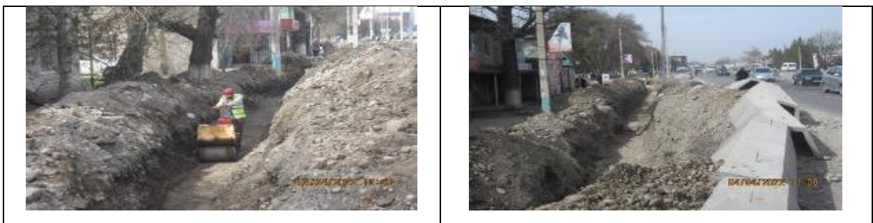
Figure 15 Installation of roadside culvert ditches at 7.4 km section
