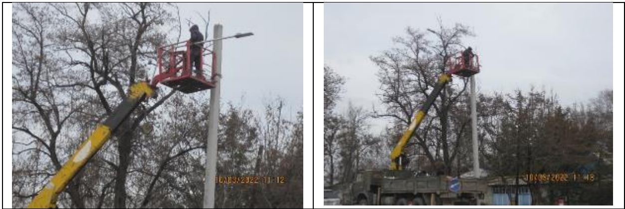
Figure 8 Street lighting works. Installation of lamps
