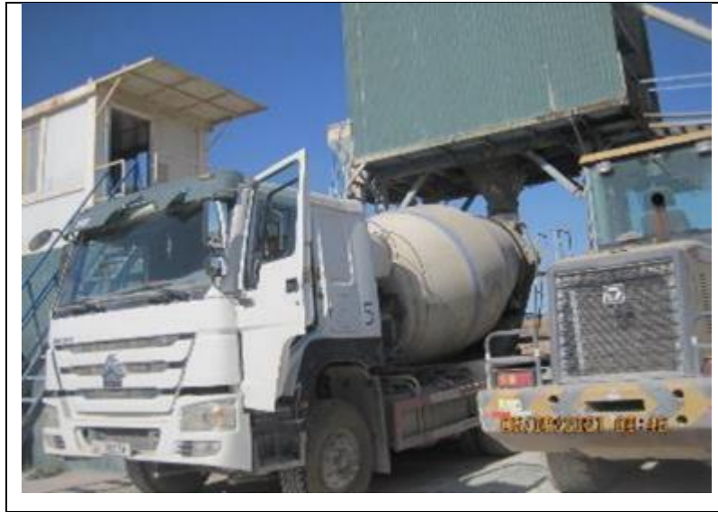
Figure 41 Refueling of concrete mixer trucks
