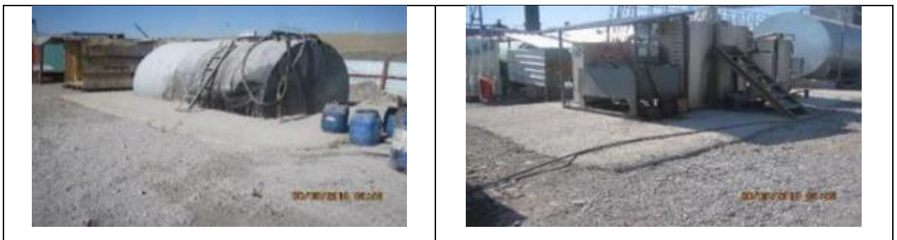
Figure 37 Impermeable protective coating around chemical containers.
