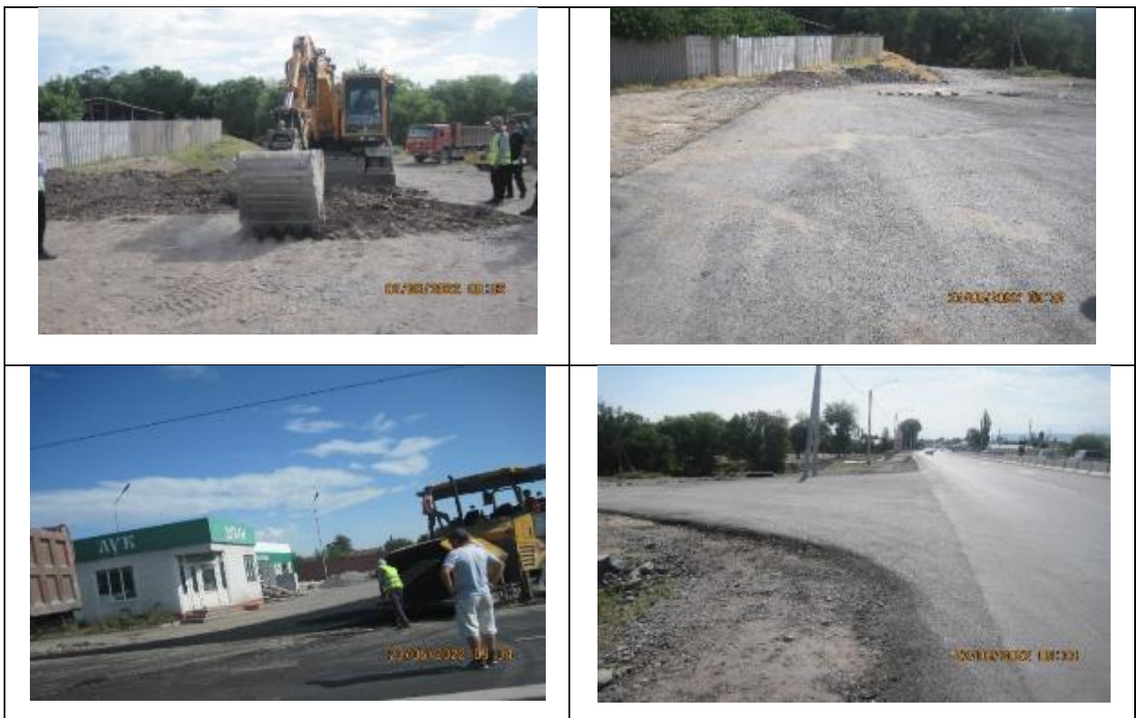
Figure 7 Laying asphalt at junctions to the streets adjacent to the road. Belovodskoe village
