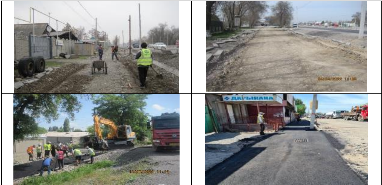
Figure 6 Construction of sidewalks
