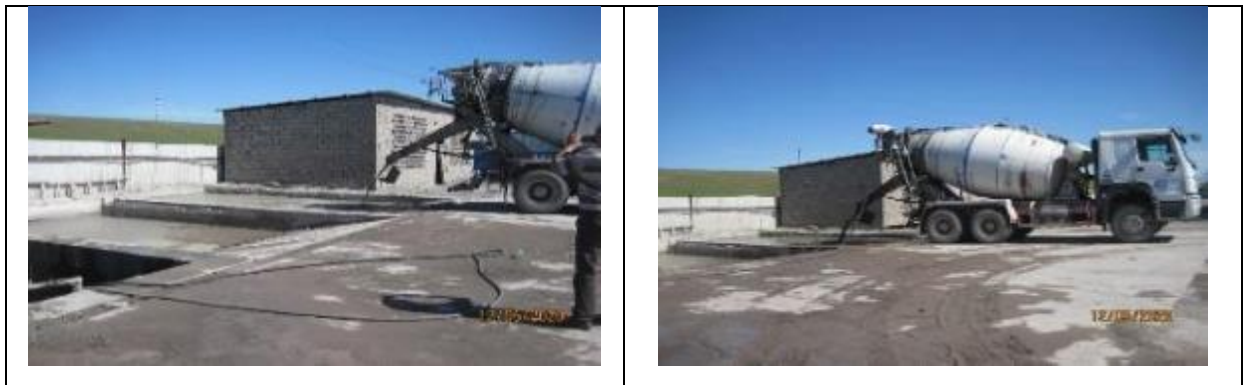
Figure 42 Washing of concrete mixer trucks.
