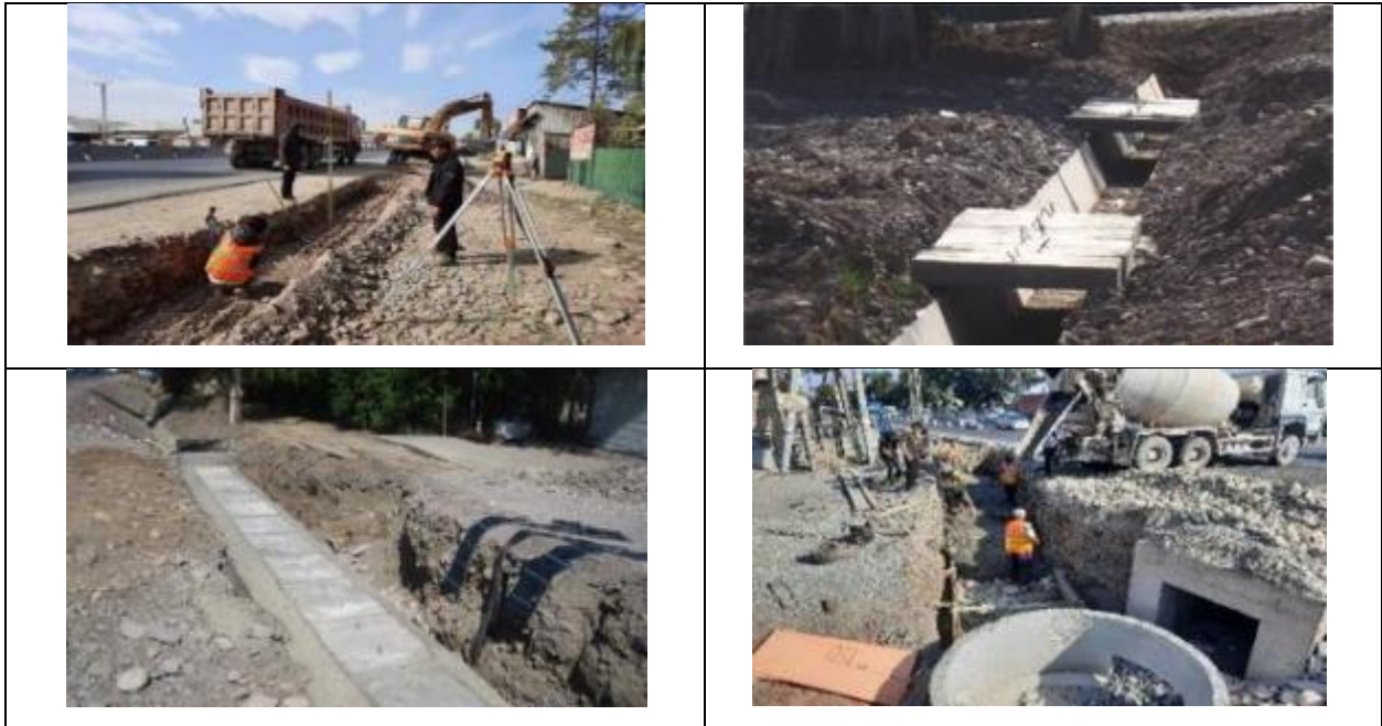
Figure 5 Installation of roadside culvert ditches and crossings to private houses and streets adjacent to the road
