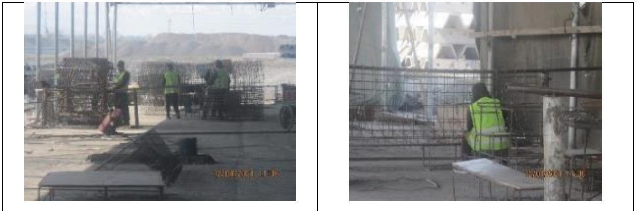
Figure 40 Production of reinforcing welded meshes, frames for the production of reinforced concrete structures
