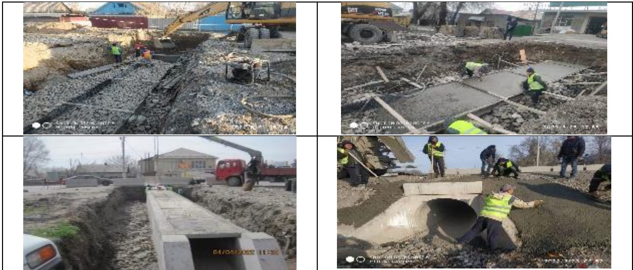
Figure 14 Construction of culvert pipes
