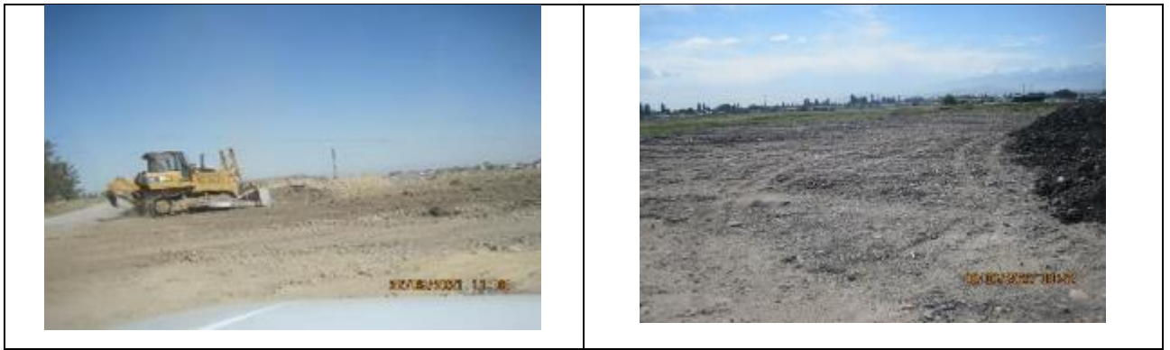
Figure 54 Storage and levelling of unsuitable soil for further use in the village of Voенно-Antonovka.
