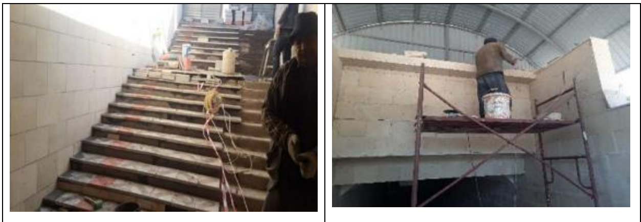
Figure 9 Completion of construction works in underpasses
