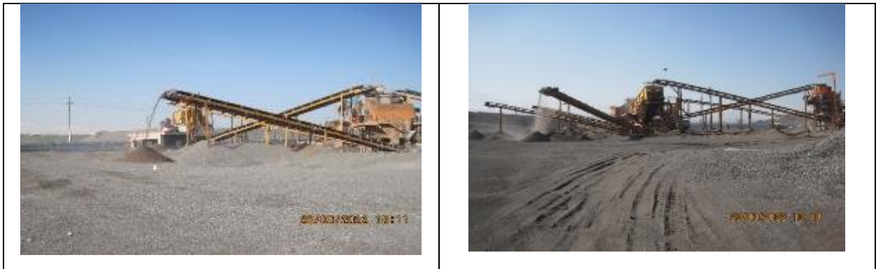
Figure 20 Stone crushing plant.
