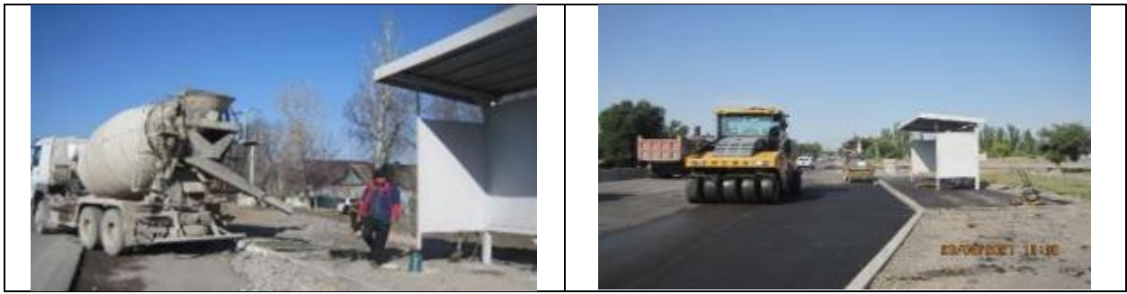
Figure 3 Asphalting of bus bay areas.
