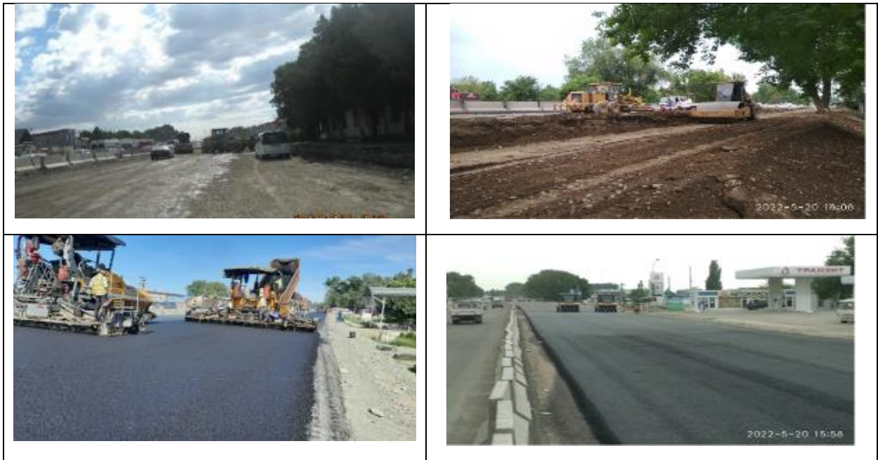
Figure 13 Rolling, soil compaction, and asphaltting of the roadbed at 7.4 km section.
